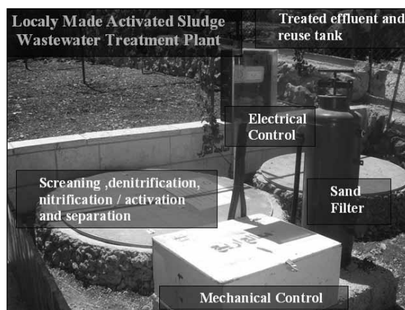
Figure 2. Description of the different components of a locally made onsite wastewater treatment system(ARIJ, 2005).
